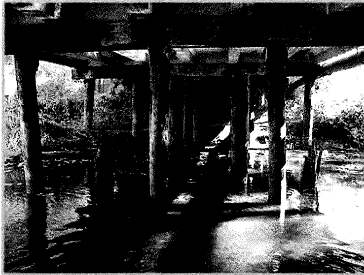
This Bridge on Friday Creek is typical of our channel beam girders supported by timber piles and caps.
